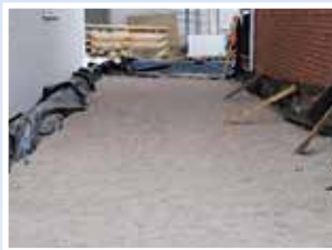
2. Lay and compact 2-6 mm clean bedding stone
