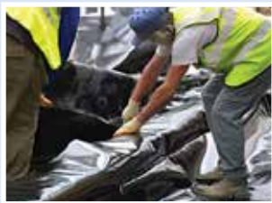
1. Install welded membrane
