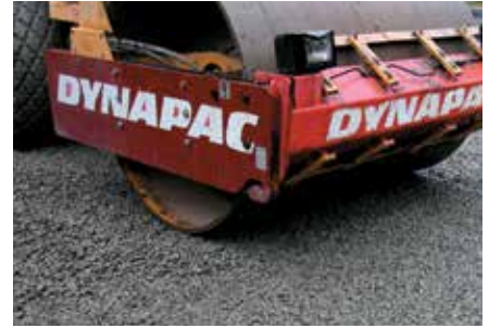
3. Compaction of the lower Sub-base.
