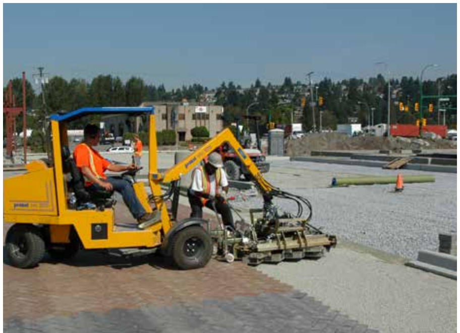
9. AquaPave® is placed using mechanical laying equipment, this can increase production to 8,000-10,000 sq. ft. per day with a standard crew.
