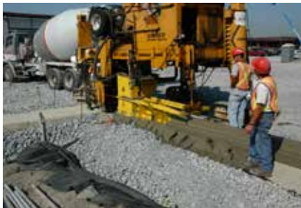
4. Paver restraints are placed.
