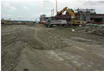
1. Excavation of sub-grade, removing any organic material.
