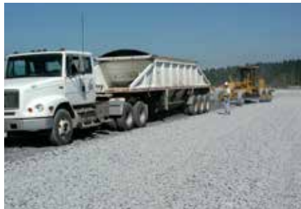
5. Clear crushed open-graded aggregate upper Sub-base is placed.
