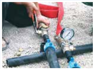
4. Pressurize and system check
