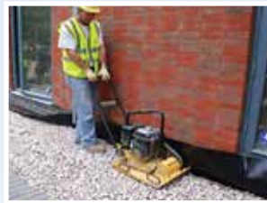
6. Compact for laying course
