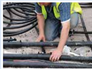
3. Install the geothermal horizontal collector pipes
