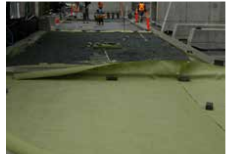
6. Placing the Inbitex® geotextile.
