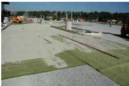
7. Inbitex® is placed followed by the 5 mm clear crushed open-graded Bedding Course .
